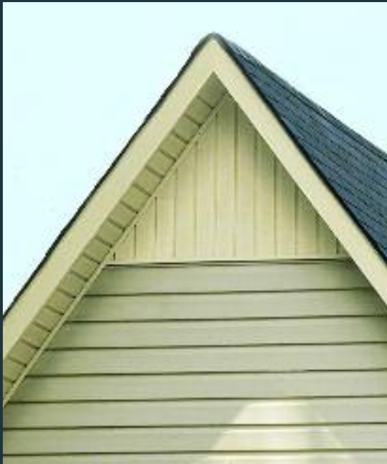
Solid panels create striking accents at entrances and gable ends.
